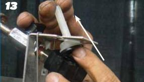
Put Diaphragm on top of Stem Assembly.
